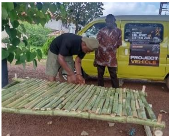
Plate 9. The researcher constructing Akwa from reclaimed bamboo. Photograph by researcher.
