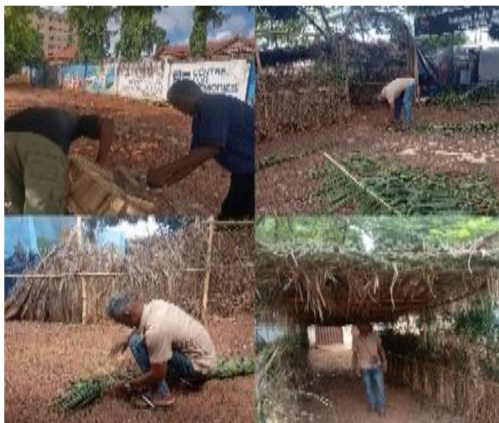
Plate 5. The researcher constructing an open-air performance space for Things Fall
