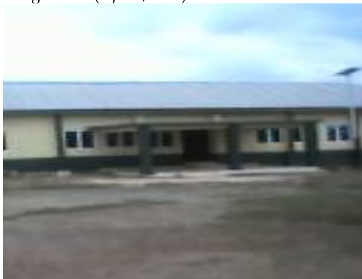
One of the renovated Buildings at the Vocational Rehabilitation Center, Emene.
