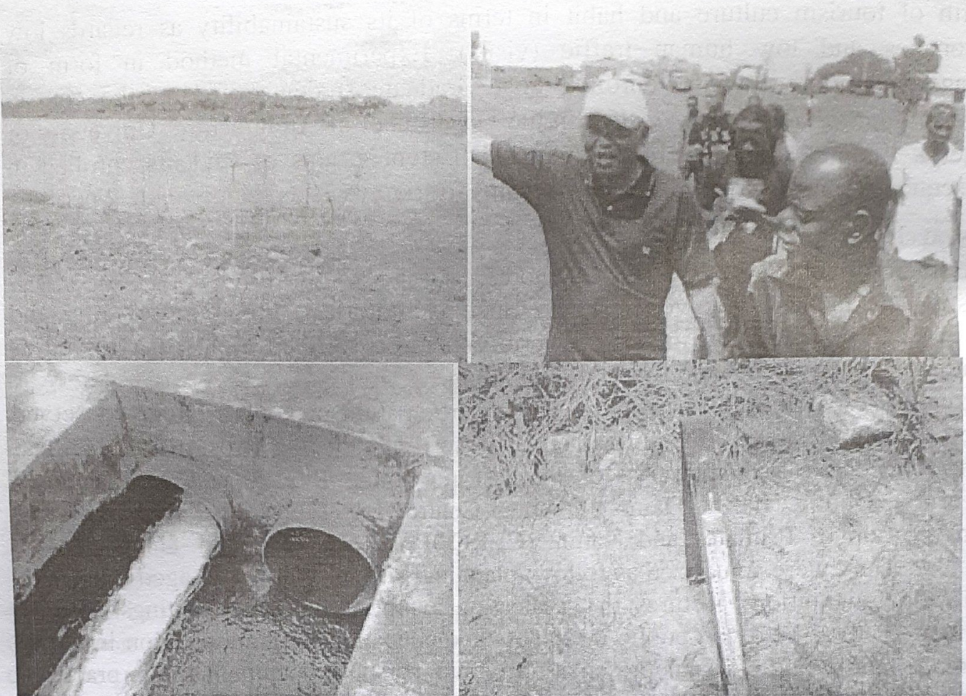
Plate 13: Dam bank, showing Rip-Rap, team on tour, valves and earth thermometer buried 5cm Source: Authors' (Field Trip) 2010
